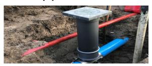
Innovative plug and play solution to place sensors into existing pipe networks
